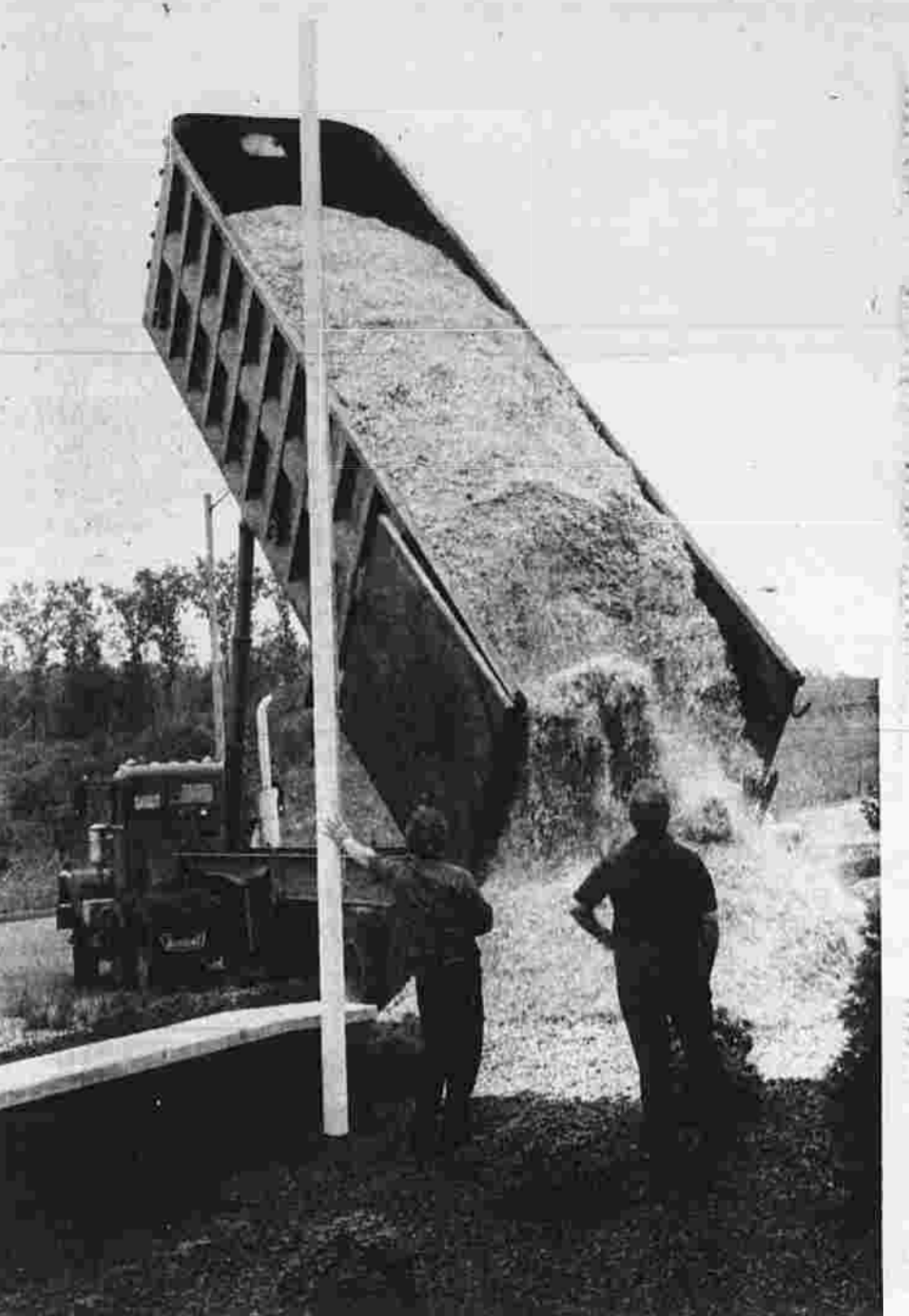
That's some load of woodchips being dumped on the area in front of Red-Lee Metal Finish Co. at Sheldon Rd. Watching the operation are Joseph Fournier, left, president of Red-Lee; and Roger Vorsine. (Herald photo by Dunn)
